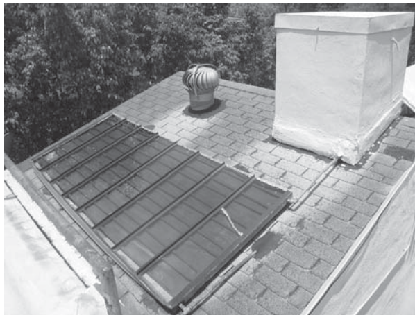
Figure 1.28 A Day-and-Night solar water heater in Florida. From 1920 to 1941, more than 25,000 solar water heaters were manufactured and installed in Florida. After 80 years, thousands of them are still working. The photo, taken by the author in Miami in August 2010, is a solar water heater installed in 1937. The insulated water tank is disguised as a chimney. Even with a broken pane, it is still working properly.
